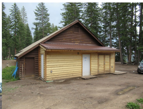
Utility room on back of dining hall
